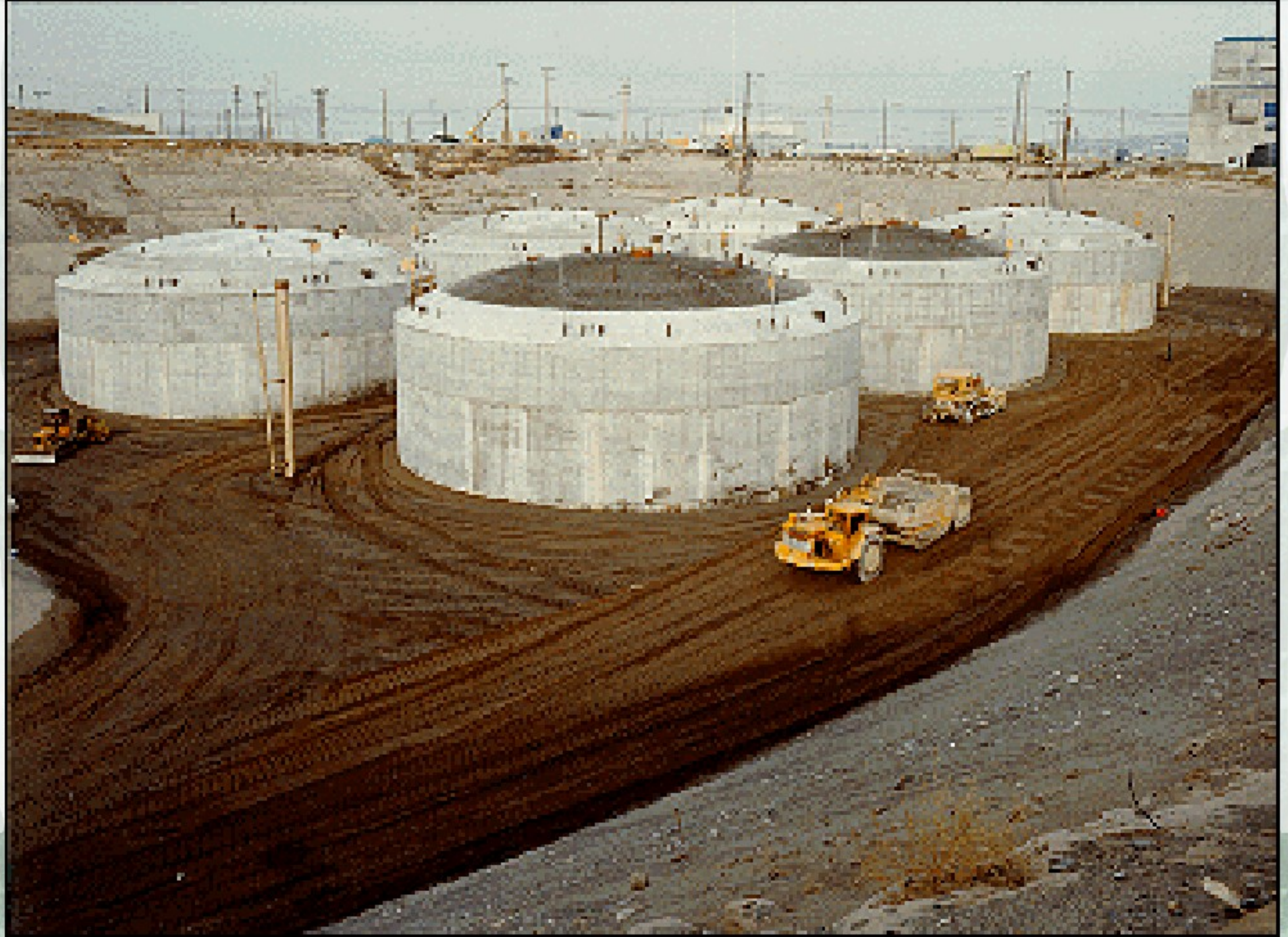
Tanks at Hanford
